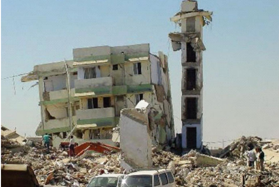
Fig. 8.1 Damage predominantly due to structural inadequacies observed during the 2001 Bhuj earthquake
