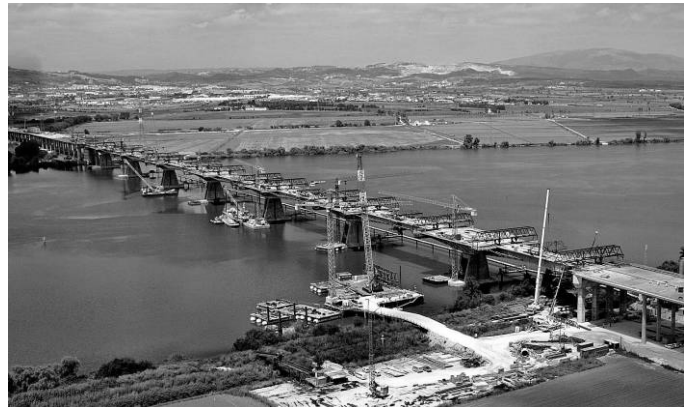
Figure 11. Lezíria Bridge: construction stage in May 2007.
