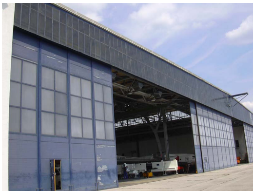
Figure 4. Long side of the building in Fig.2
